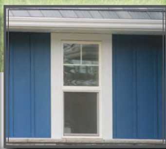
Soffit, Fascia and Trim
